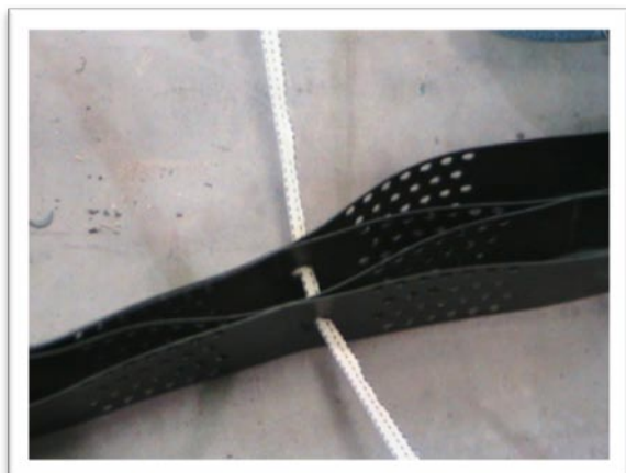
5. Pull the tendon completely thru the EnviroGrid.
