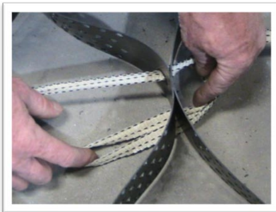
9. Feed loop under EnviroGrid.
